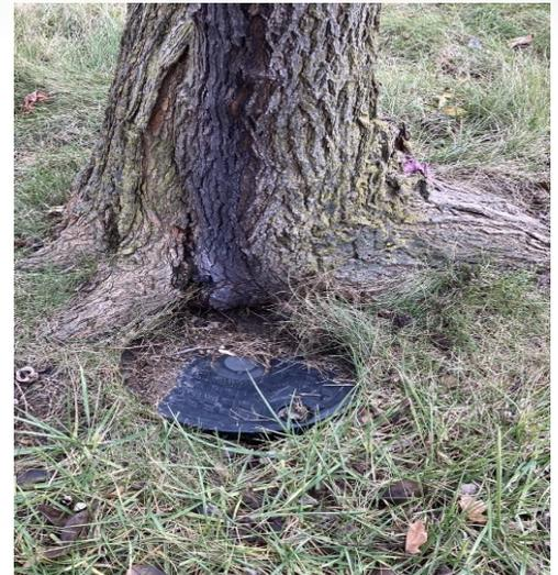
Do not block access to the water meter pits with landscaping timbers or concrete pavers, bushes, flowers or shrubs. When planting trees, make sure that they are not placed close to water meter pits.
