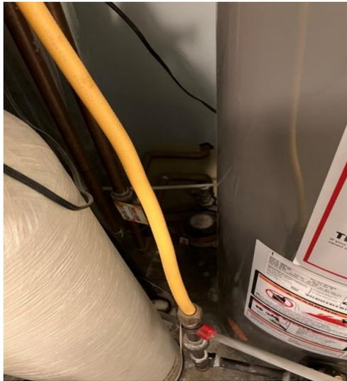
Please do not install any appliances or place any hard-to-move items where our service technicians cannot easily reach the water meter to perform that work. As the picture illustrates, the water meter is blocked by the water heater, water softener, and gas line preventing access to replace water meter when necessary.
