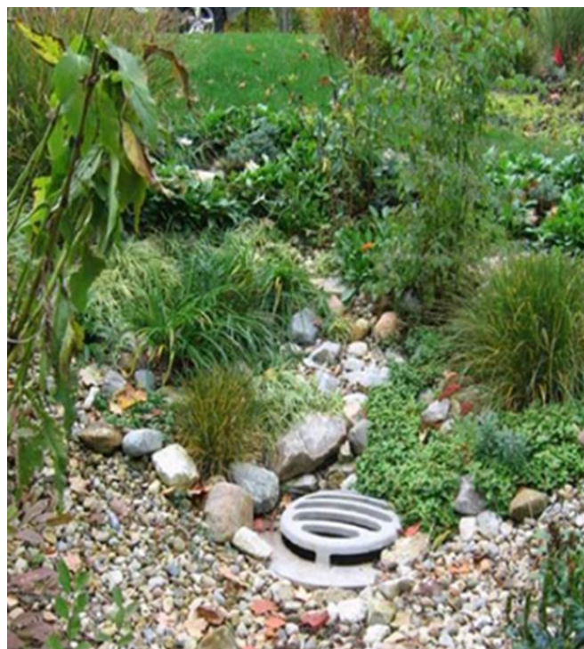
Example of rain garden with overflow structure.
